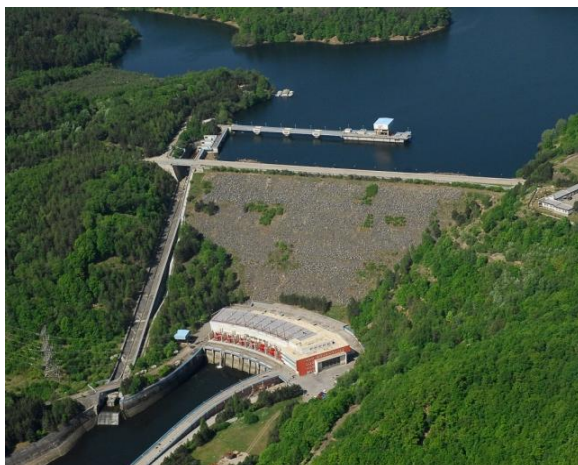
Figure 1. Pumped-storage power plant Dalešice (Czech Republic) ( http://www.cez.cz )
