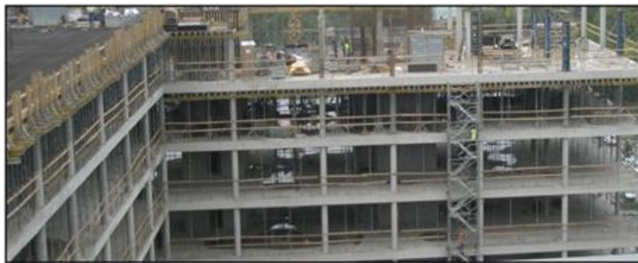
Figure 3. The load-bearing monolithic reinforced concrete structural system of the monitored structure
