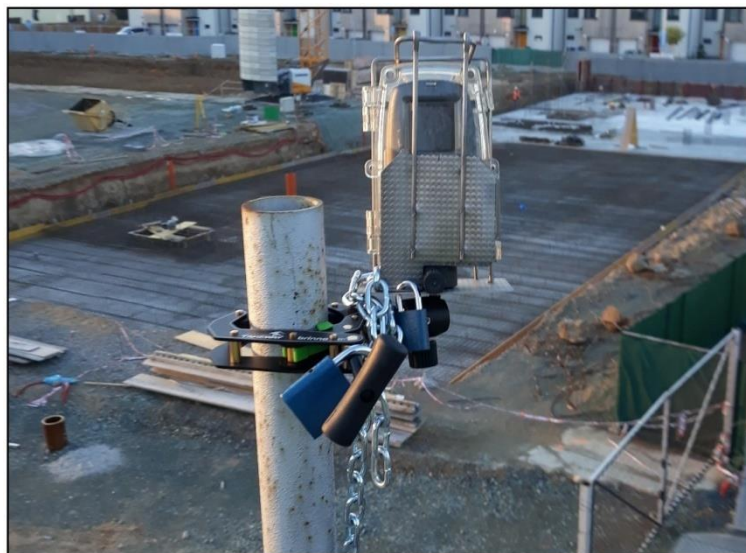
Figure 7. Monitoring device in a protective cage
