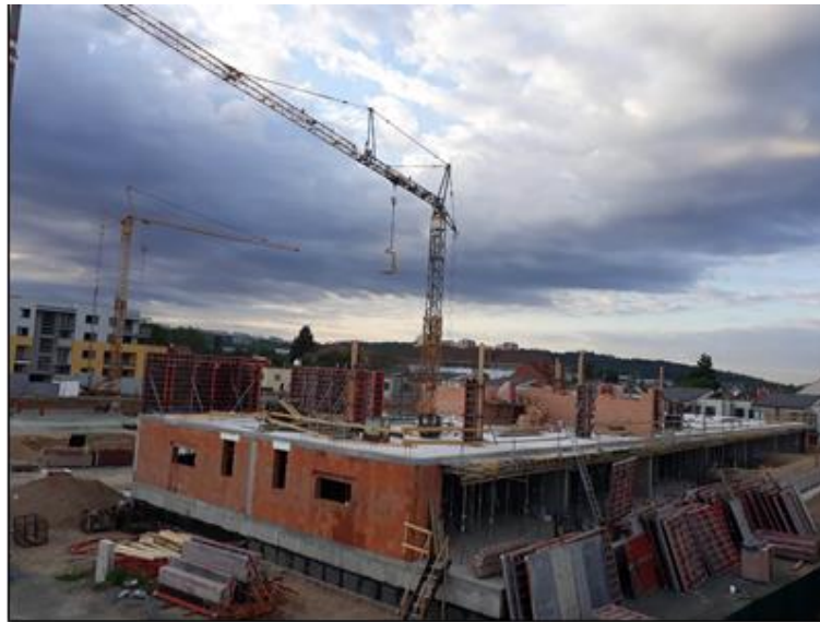
Figure 4. Construction of the monitored apartment building
