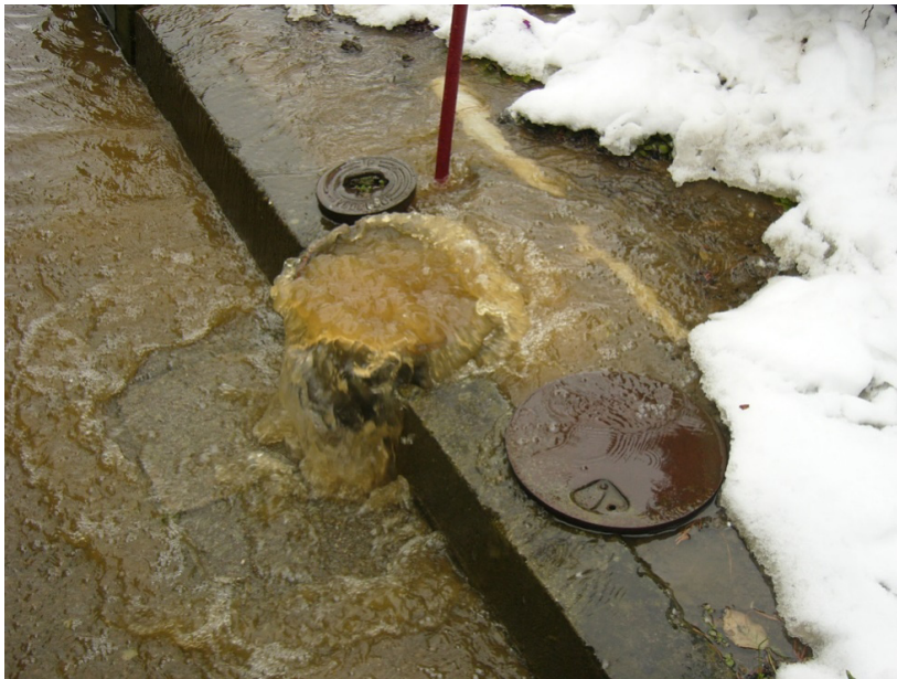
Fig. 1 Case study Kateřinice – water main flushing
