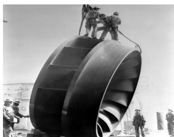
obr. 3.5 Rotor Francisovy turbíny
