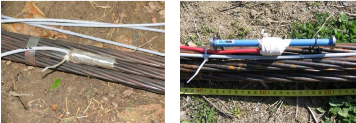
Fig. 1. (a) the foil strain resistance gauge stuck on the tendon; (b) the Vibrating wire strain transducer fixed to the tendon.
