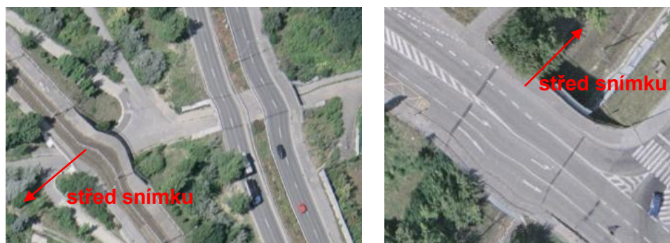
Obr. 54: Deformace na mostech
