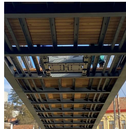
Figure 4 Footbridge over the Svitava River in Bílovice nad Svitavou, Czech Republic, equipped with a tuned mass damper KGF (Nečas, 2023)
