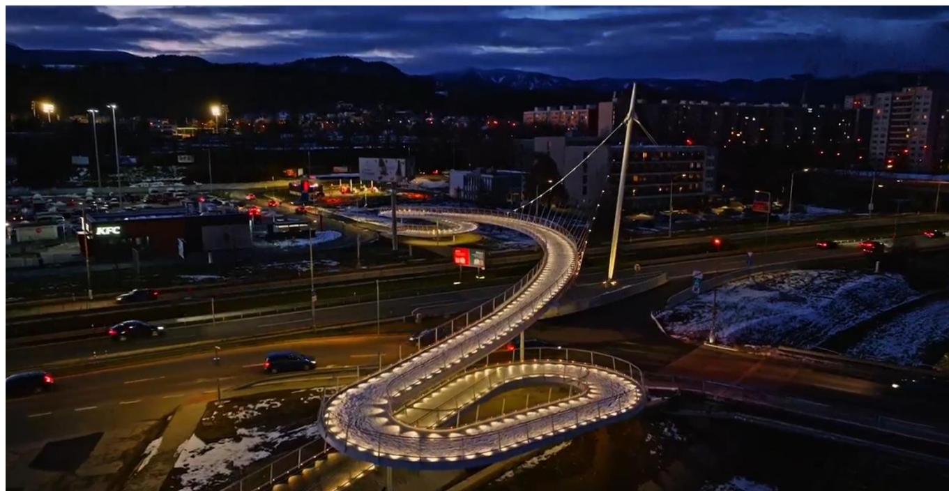
Figure 5 Bicycle bridge over the R1 expressway in Banská Bystrica, Slovakia (Ingsteel, 2024)
