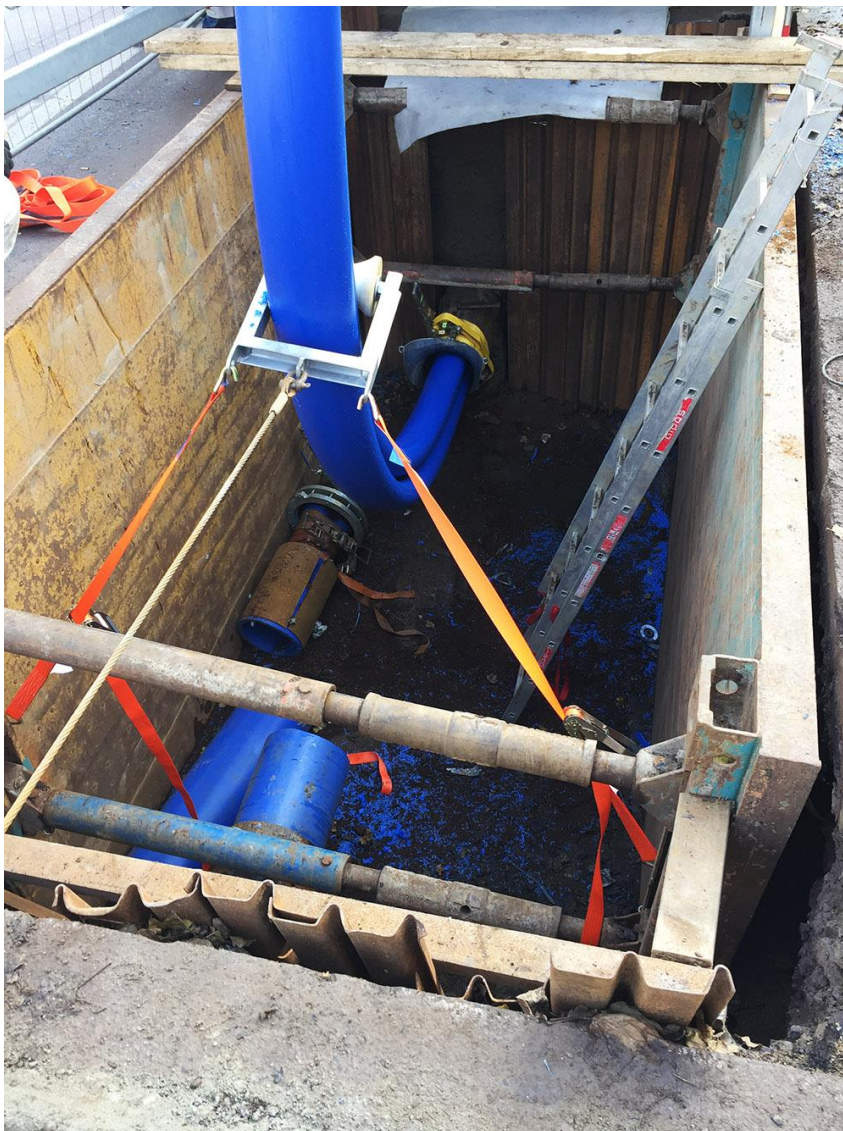
Obr. 4.9. Technologie Compact pipe [24]
