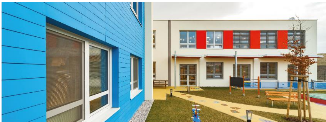
Figure 1. Ventiladed facade, application of cement fiber boards 0
