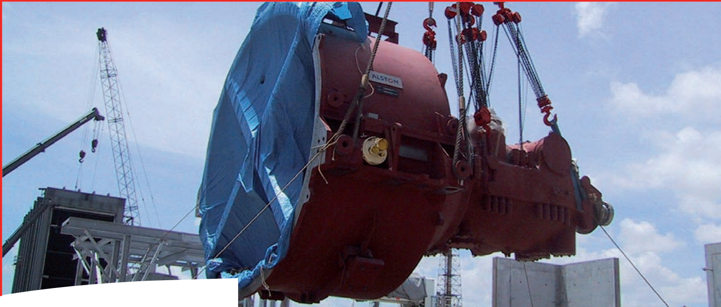
Completely shop-assembled 200 MW cogeneration steam turbine at site installation
