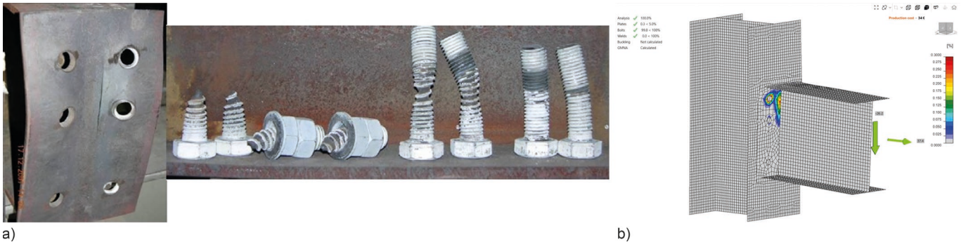
Fig. 14 Deformed shape of the connection at 650°C: a) test and b) CBFEM
