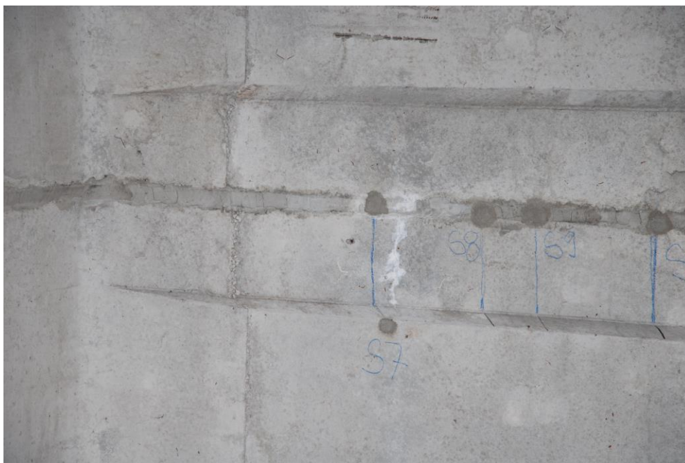
Obr. 3.20: Spára mezi lamelami [25]
