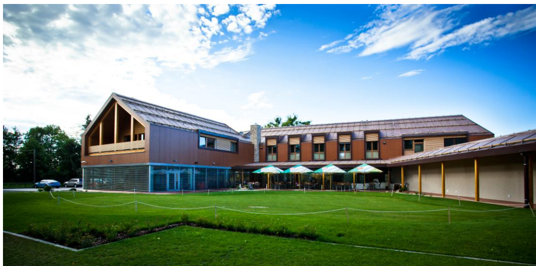
Obr. 8: Budova Silesia Golf Resort II.
