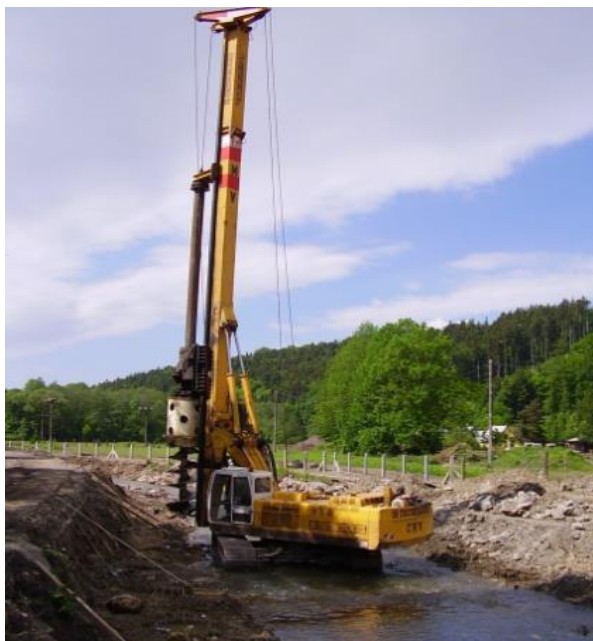
Obr. 6.12 Vrtná soustava pilot VMV TH 15-50 [31]
