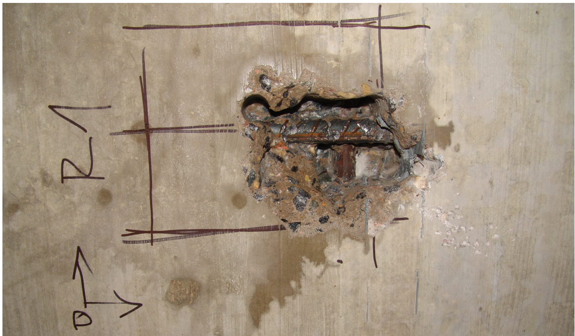
Obr. 22: Detail sekané sondy R1 [F]
