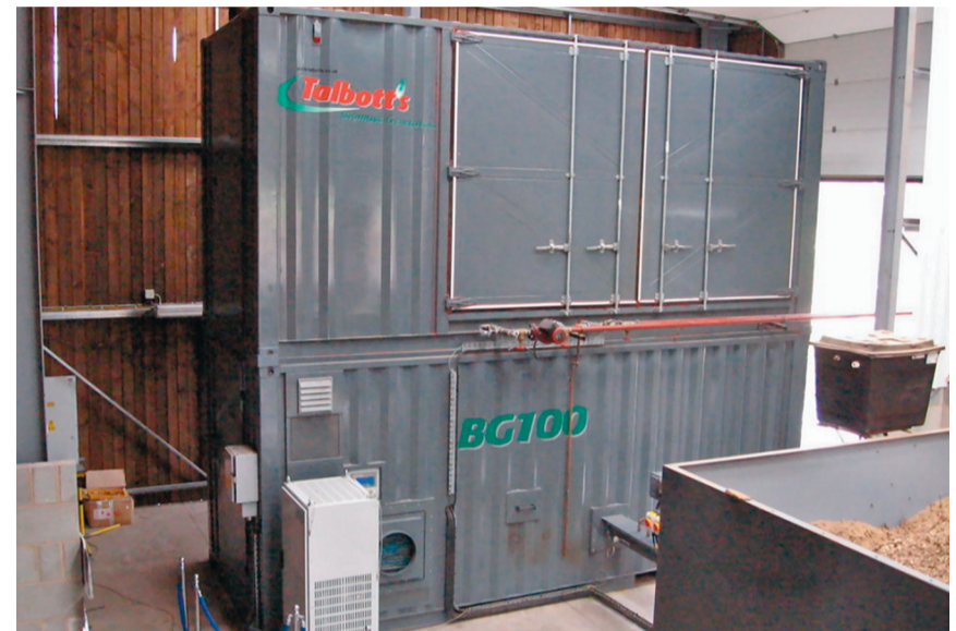
The containerized system of the BG100. To the right, the wood chip fuel bunker and supply.
