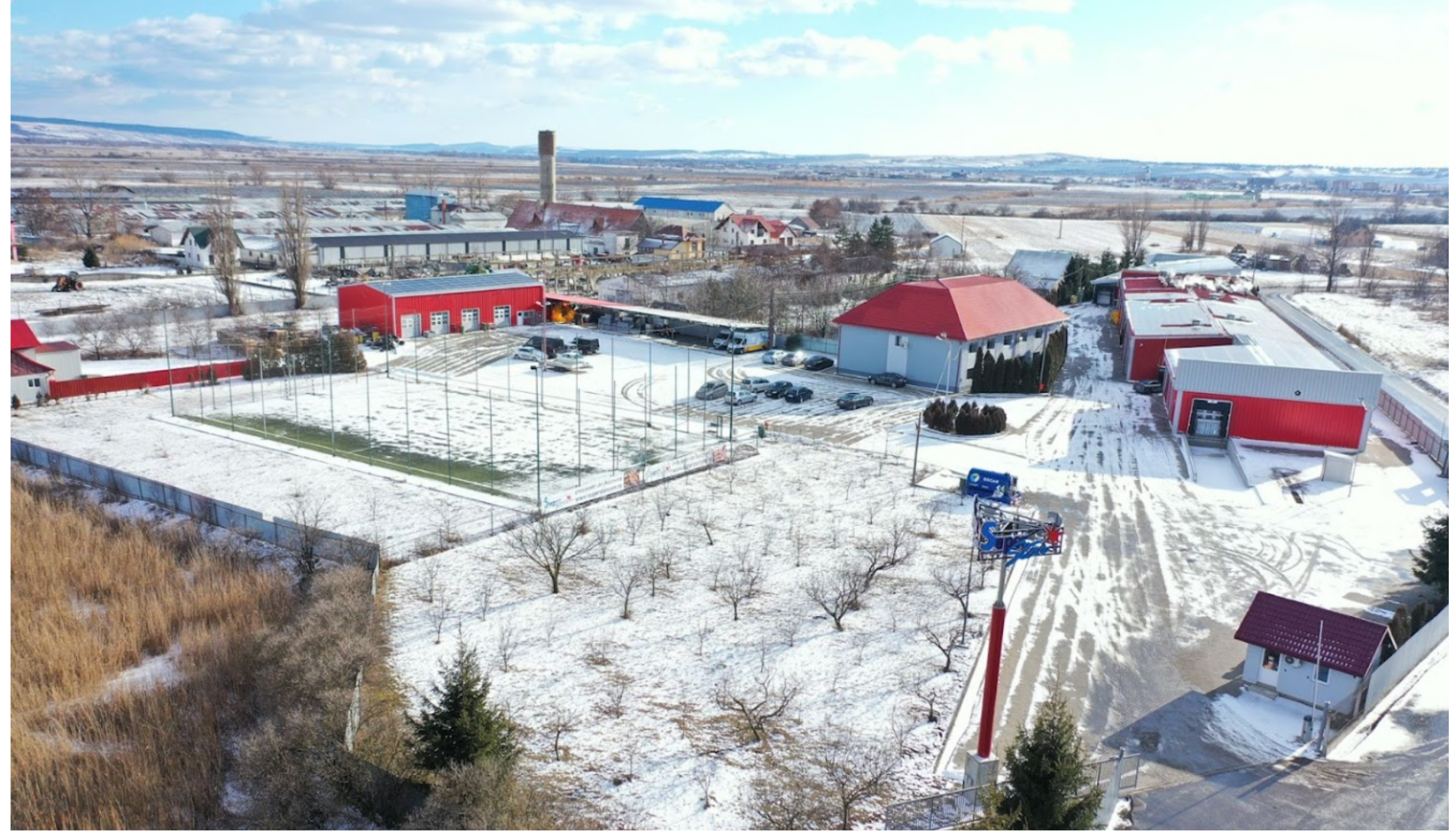
Aerial view of existing site.
