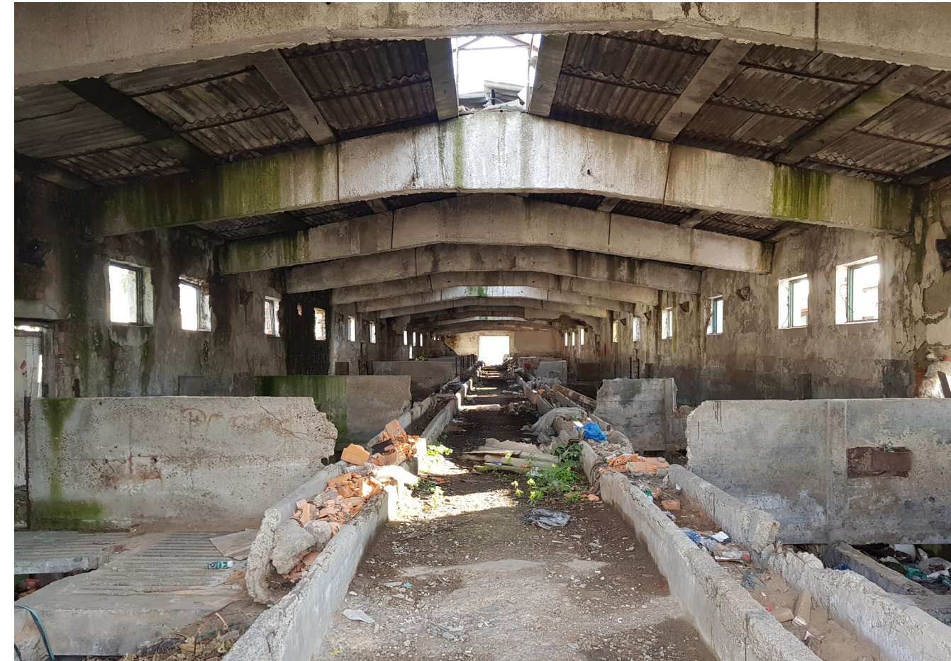
Internal view of concrete beams, partition walls and roof substructure.
