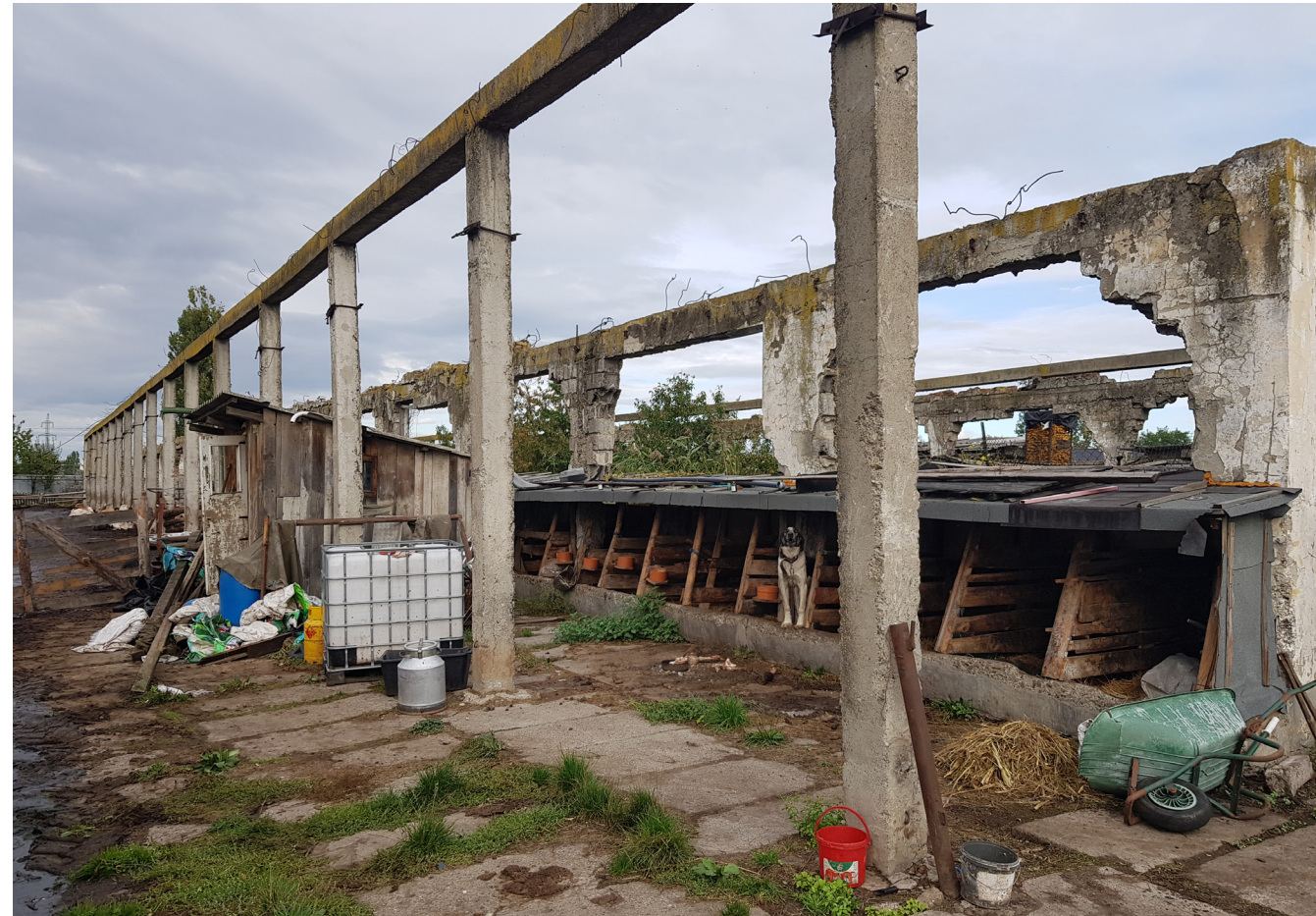
External view of structural grid without partition infills and roof.
