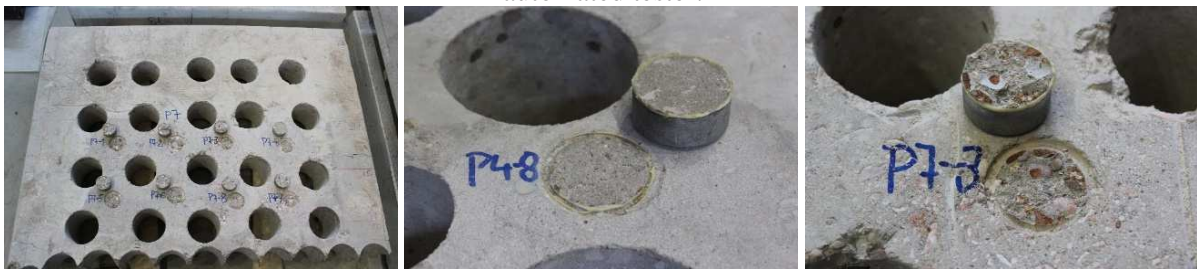
Figure 2. Pull-off bond strength test: a) selected panel (panel P7 loaded with 1000°C) after performing the pull-off test, b) detail of testing point P4-8 on the thermally unloaded panel P4 after performing the pull-off test, c) detail of testing point P7-3 on the thermally most loaded panel P7 after performing the pull-off test.
