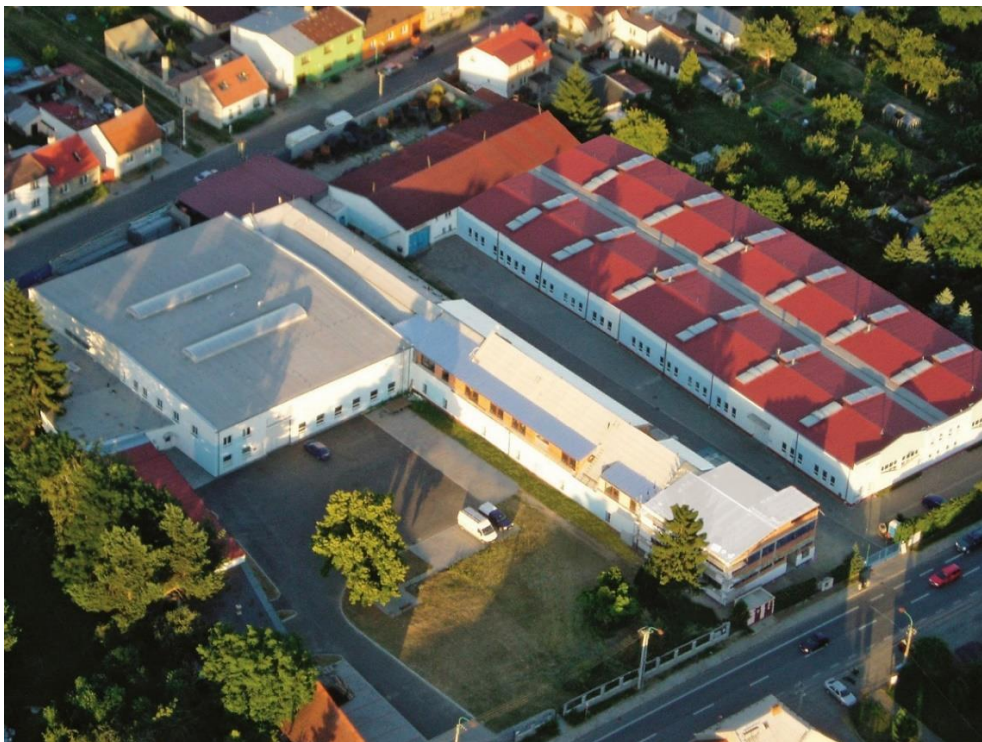
Obr. 2 Prostory ABO Valve [3]
