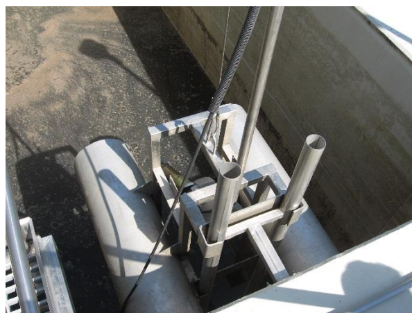
Obr. 6.2-24 ČOV F - Systém Triton
