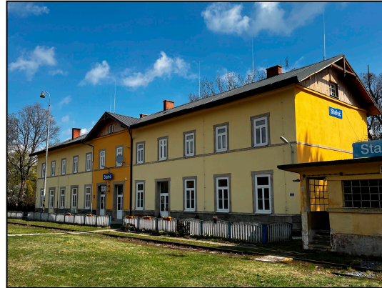
Figure 6. Station building in Stařeč (CR) [59].
