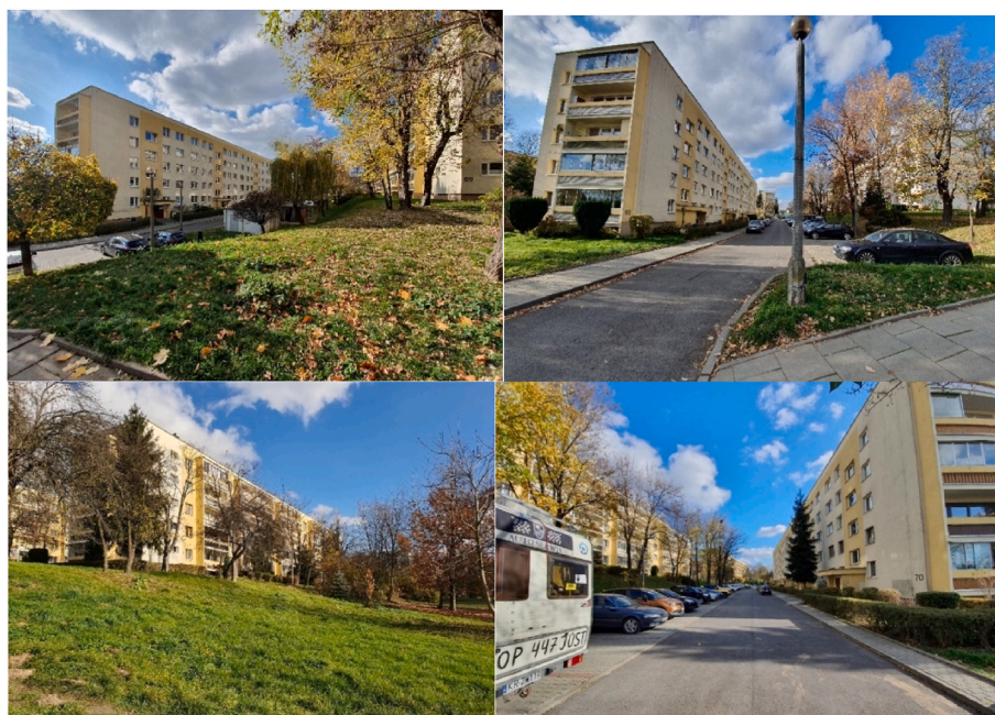
Fig. 5. Photos of the building selected for the formulation of detailed solutions and the building’s surroundings, 2021 original work; clockwise: view from the northeast; view from the east; view from the west, northern facade; view from the southeast, southern facade.
