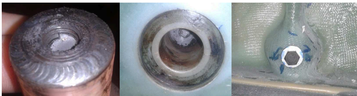
Figure 7: Root rib pin has failed. After it has been repaired, the fatigue test continued.
