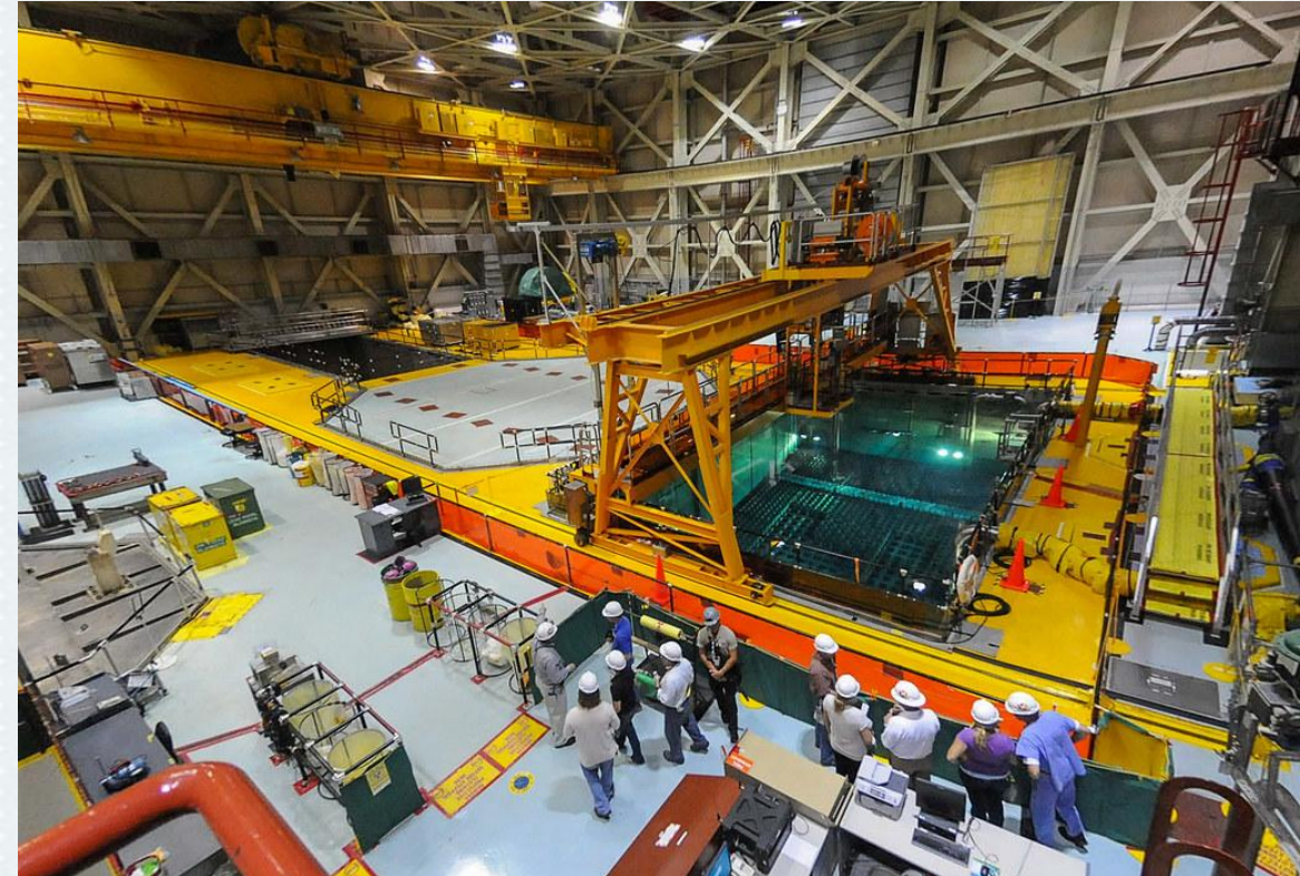
"Spent Fuel Pool of Unit 2 at Brunswick Nuclear Power Plant" by NRCgov is licensed under CC BY 2.0 .
